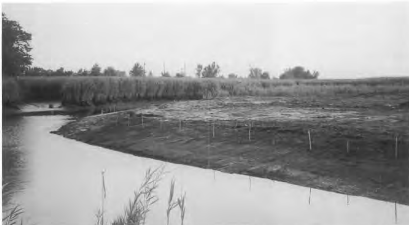
After construction at the NYS DEC Healy Avenue Restoration Site in the Jamaica Bay Watershed, June 1998
